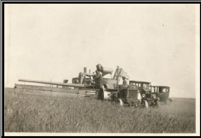
Two man straight combining operation with early Model 5 Massey Harris combine and Hart Parr tractor (no power take off or hydraulics!)
