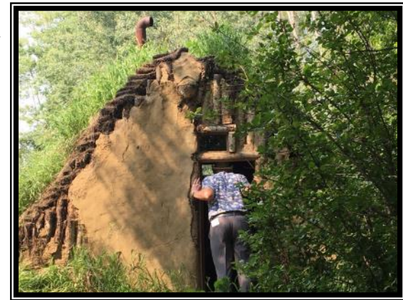
A replica of an earthen hut, also known as a semlin or sod house
