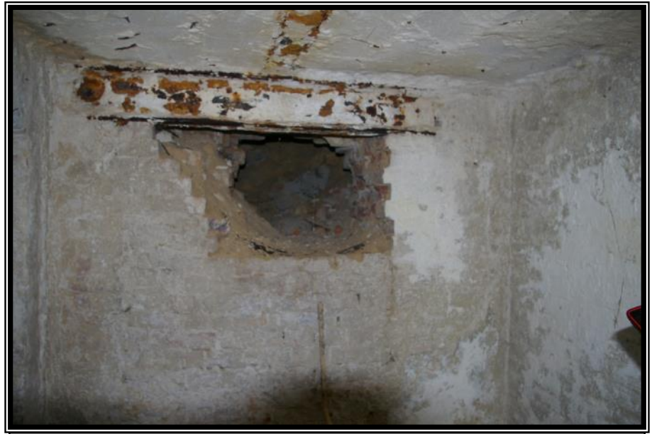
Tunnel entrance in the basement of the old Credit Union building, showing an opening in the bricked-over section.
