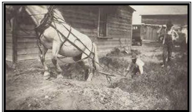
Horse and scraper digging a basement
