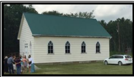
Mayfair Mennonite Church with new shingles and siding, 2018
