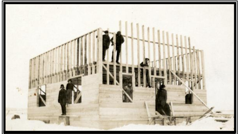
Building house on Loewen farm in Simons Valley, c.a. 1930
